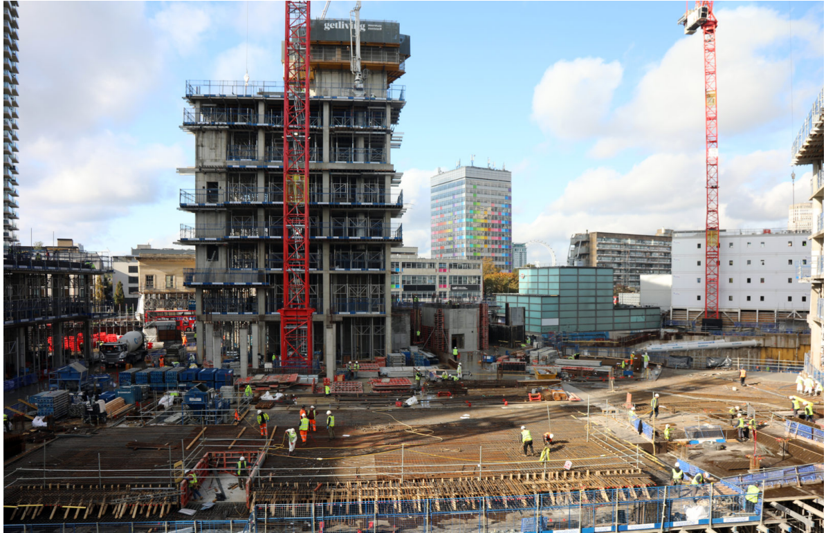
Fig. 2 Construction site, Elephant & Castle, London, 2023. Photo: David Cross.
